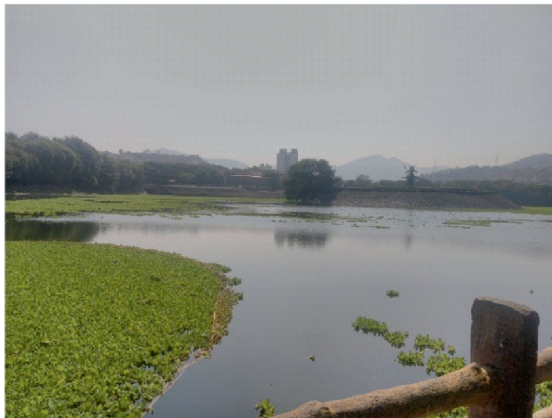
Present condition of Katraj upper reservoir
